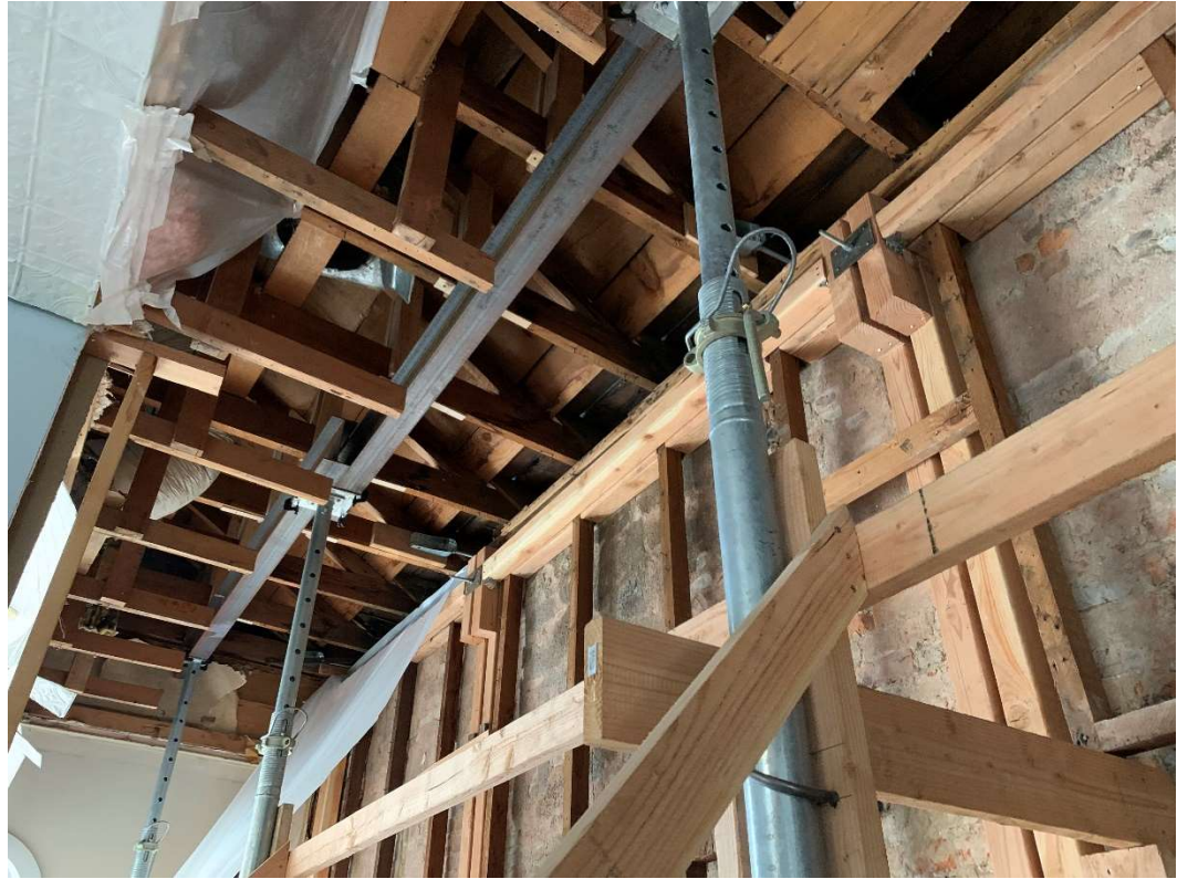
Photo #12: Company Hall Building Roof Trusses bearing on existing furring stud
