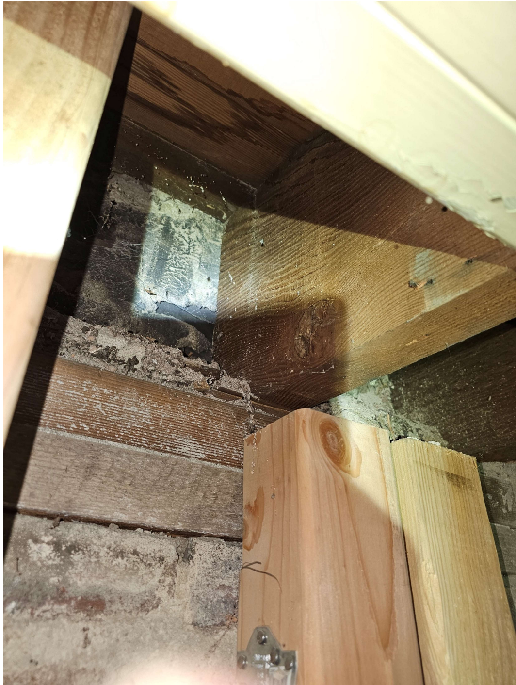
Photo #15: Company Hall Building 2 nd Floor West wall support
