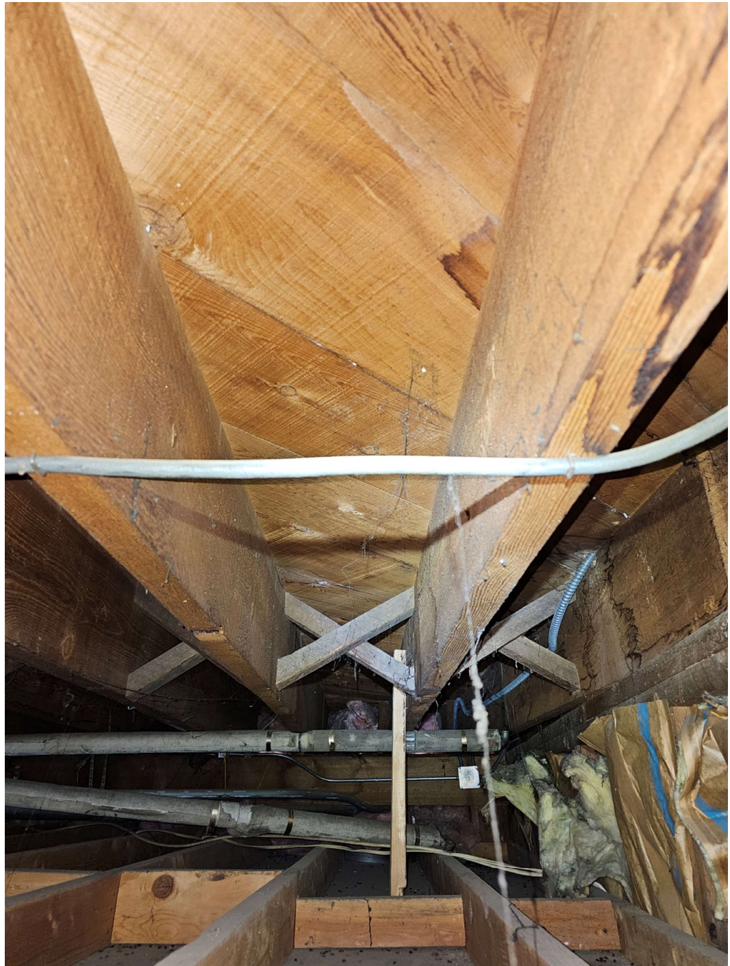
Photo #19: Emigrant Jane Building 2 nd Floor Framing
