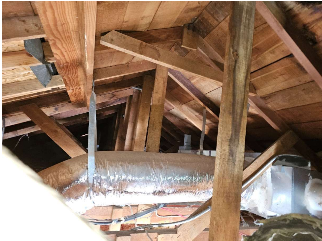
Photo #11: Company Hall Building Roof Trusses
