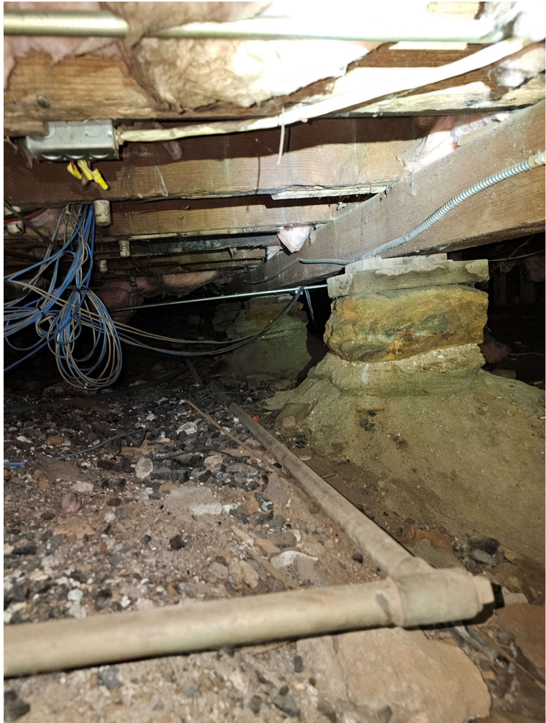
Photo #8: Crawl space view from Confidence Engine Company Hall
