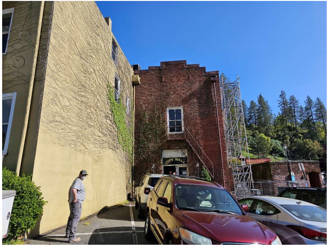
Photo #4: North Elevation (Confidence Engine Company Hall)
