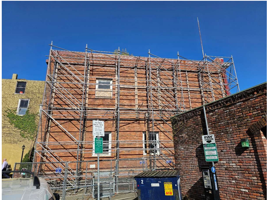
Photo #5: West Elevation
