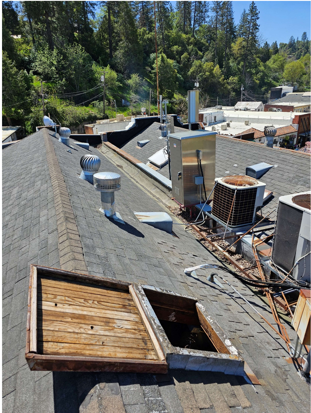
Photo #6: Rooftop View (Looking South)
