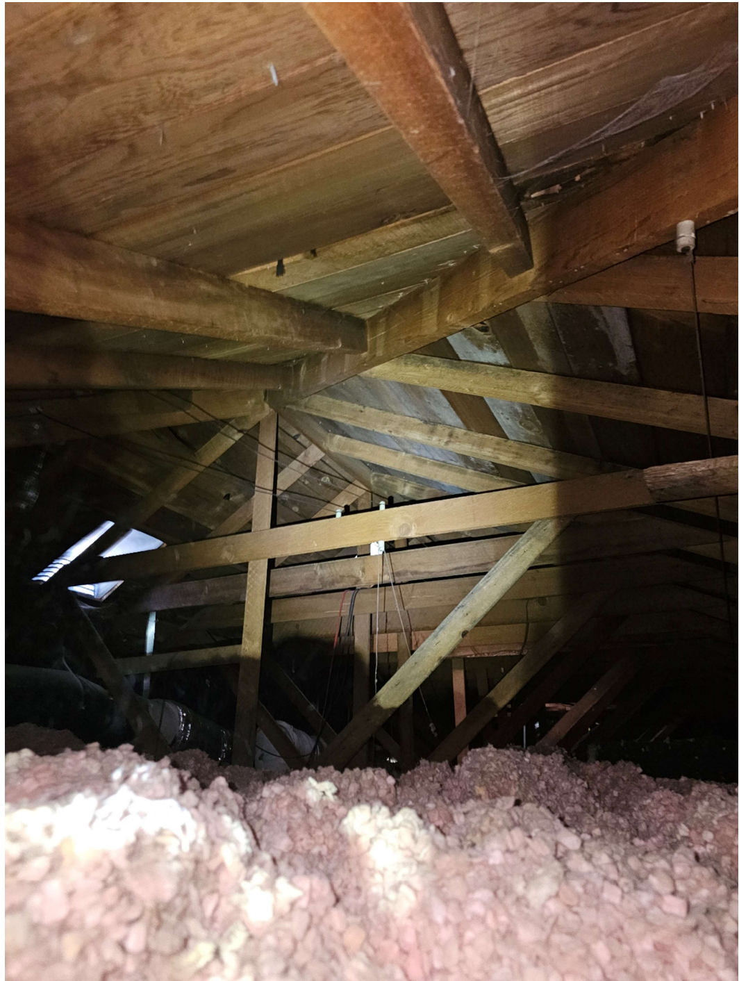
Photo #18: Emigrant Jane Building Roof Trussed Rafters
