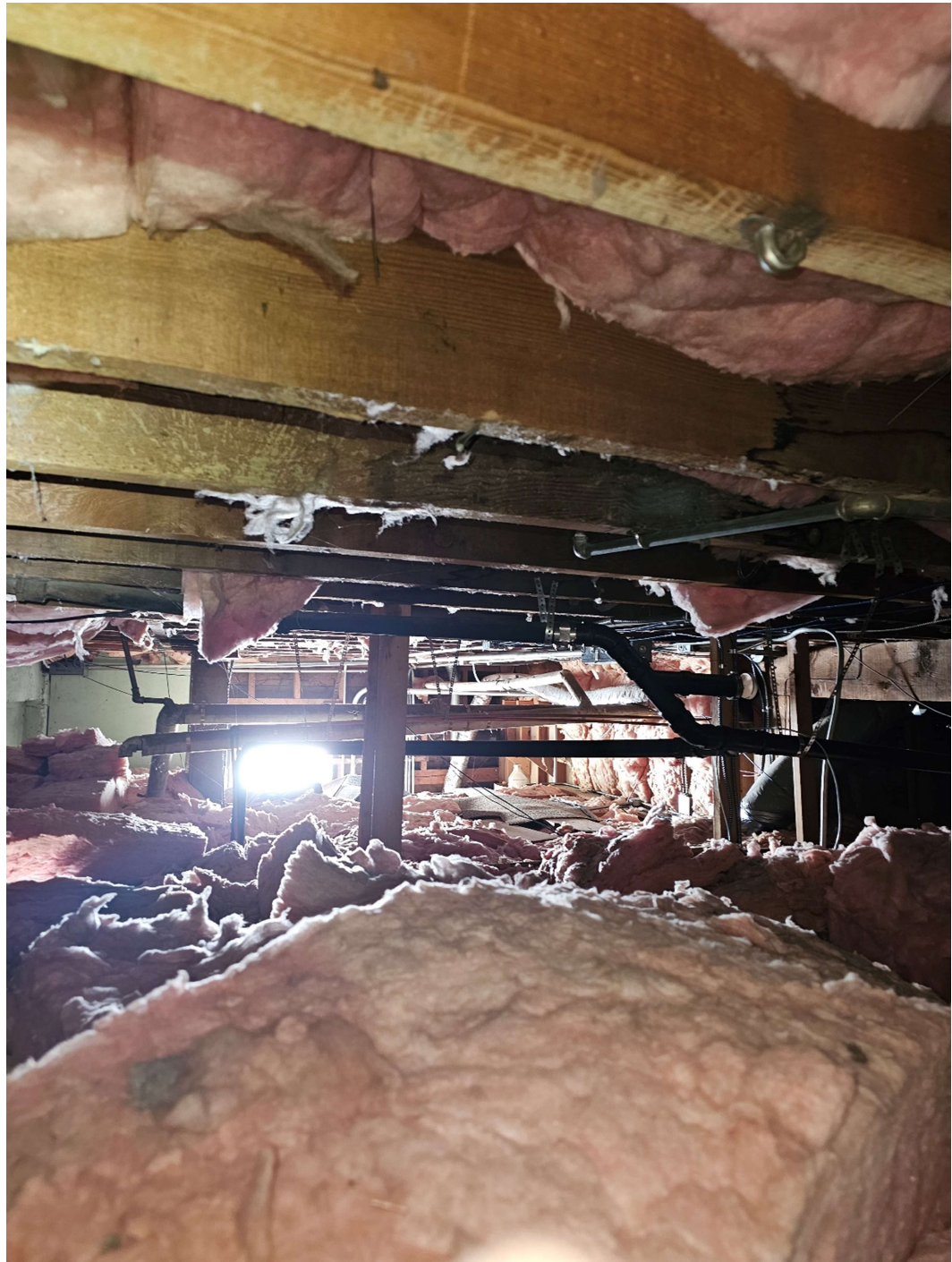
Photo #20: Rear Addition Building view of 2 nd floor framing
