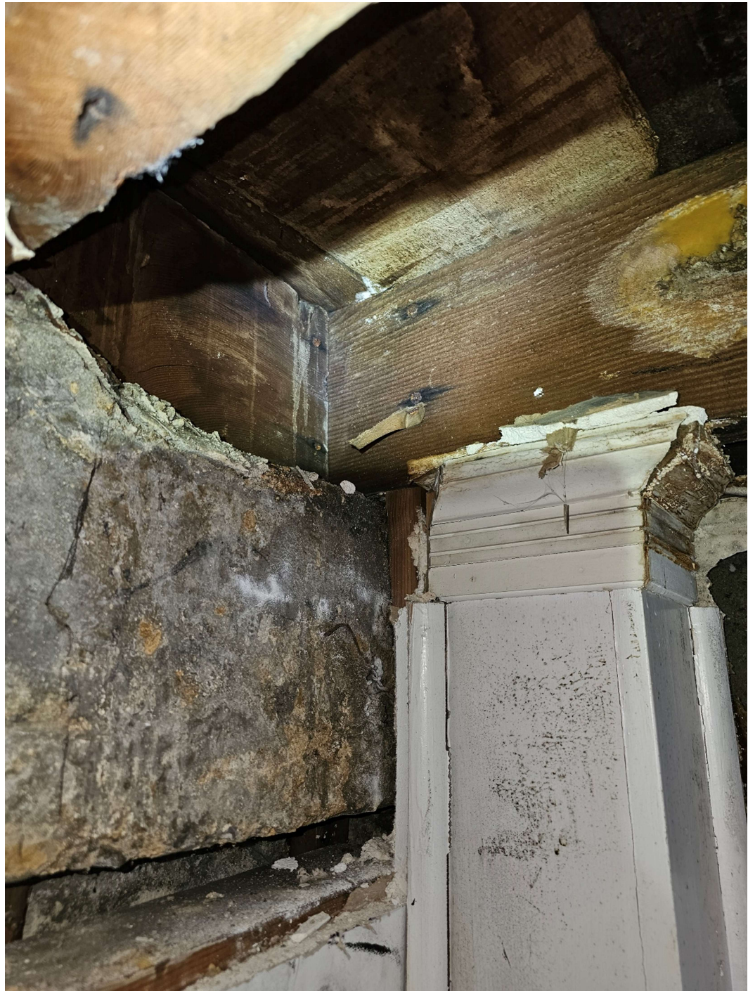
Photo #21: Rear Addition Building Roof Ceiling Framing
