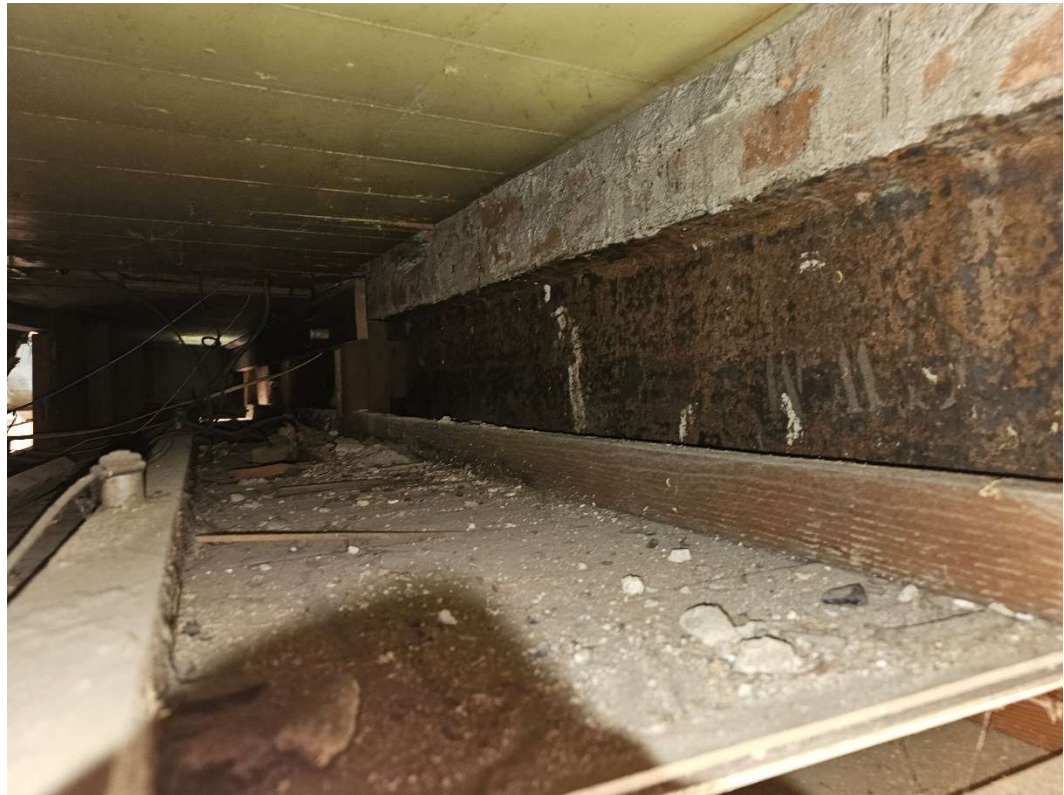
Photo #17: South Wall End Steel Beam
